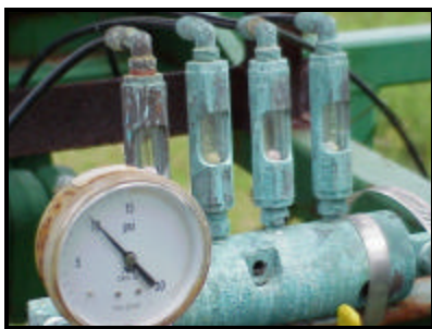
Fig. 2. Flow divider with sight glasses and pressure gauge.
