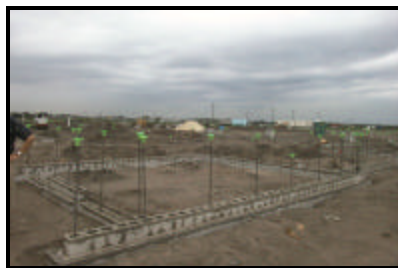
Building foundations are being completed.
